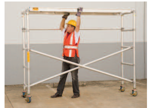
3. Install platform at desired height.
