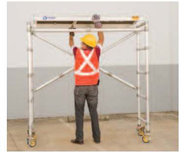
4. Install platform at desired height.
