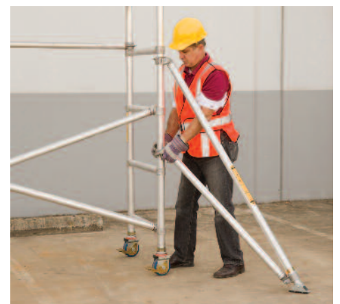
3. Before moving platform higher than 7ft. (2.1m), tie the scaffold into the building or install outrigger on each corner. Make sure each outrigger is wedged against solid pavement and that all couplers are securely fastened.
